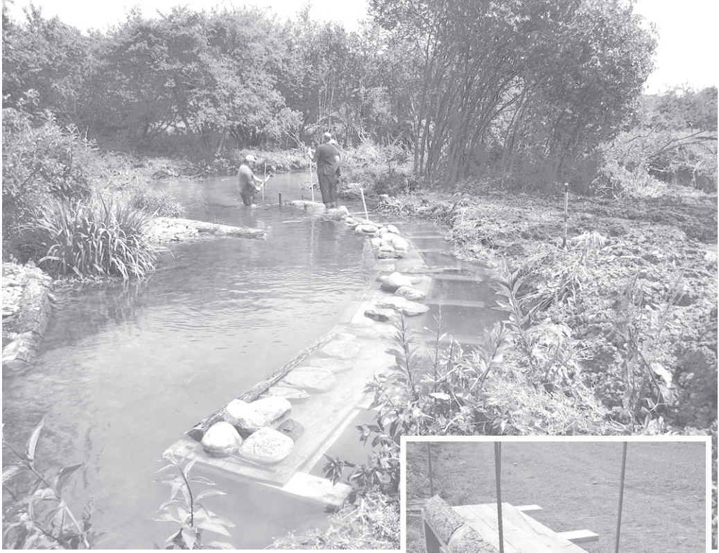
Lunkers are lined up along the creekbank, weighted down with rocks and ready to be covered. A total of 57 lunkers were placed. Inset: A lunker ready to go, complete with rebar to hold it down. Each creates an artificial undercut bank to serve as habitat for adult trout.
