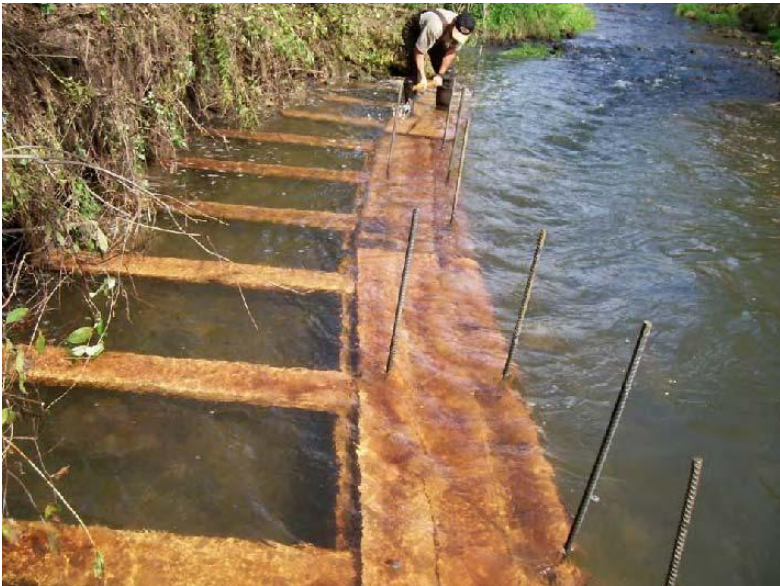
A View of Lunkers Installed in the Stream
