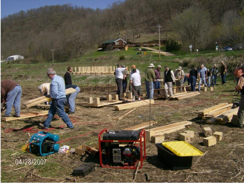
Constructing "Lunkers"
